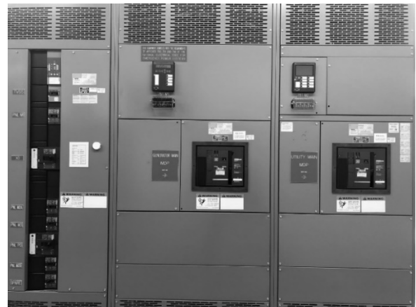
Fig. 1 Typical Service Entrance With Multiple Sources
